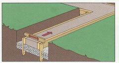
**5.** Screed concrete by seesawing a 2×4 along top edges of forms, removing excess concrete as you go.
